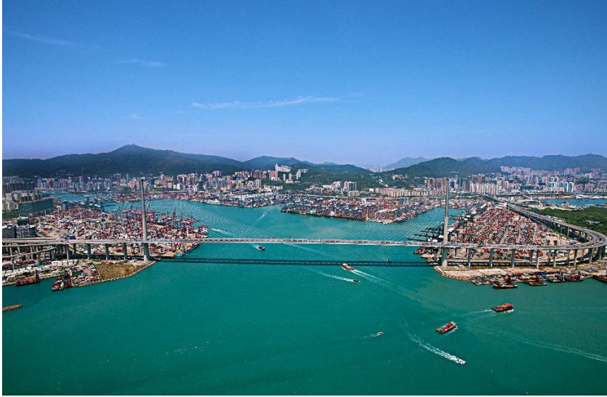
Aerial view of Kwai Tsing Container Terminals
